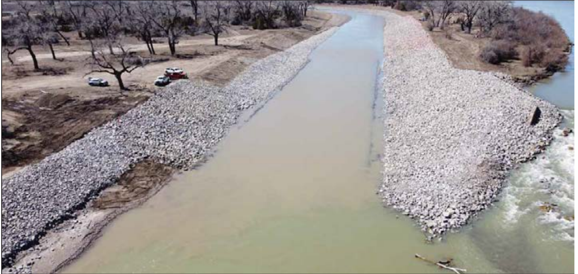
Yellowstone downstream end of bypass channel. (Photo by USACE Asset)
