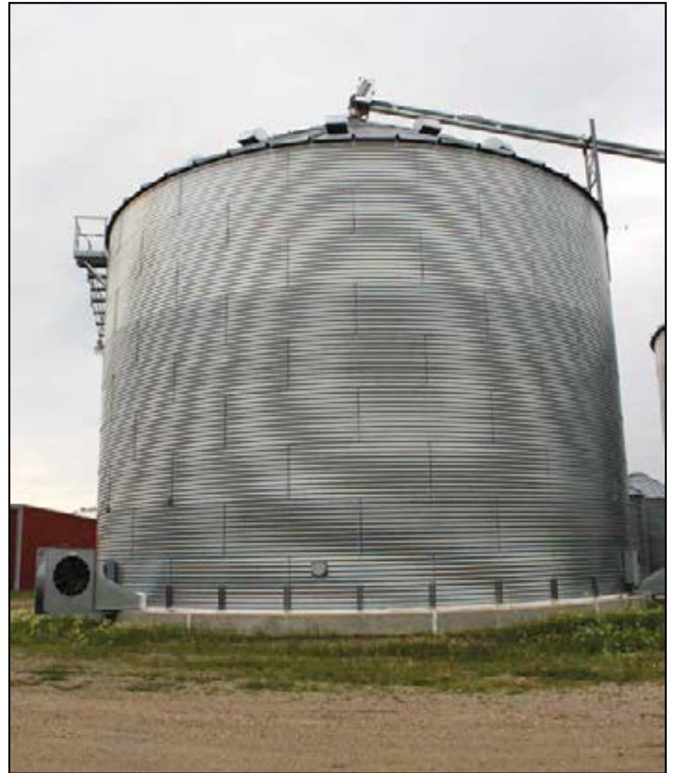
Be proactive against mold growth in grain storage by monitoring temperature and moisture. (NDSU photo)
