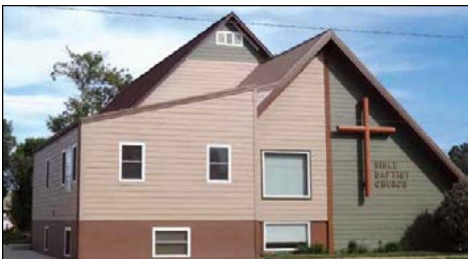
Photo taken shortly after the addition was completed in 2013. (Photo submitted)
