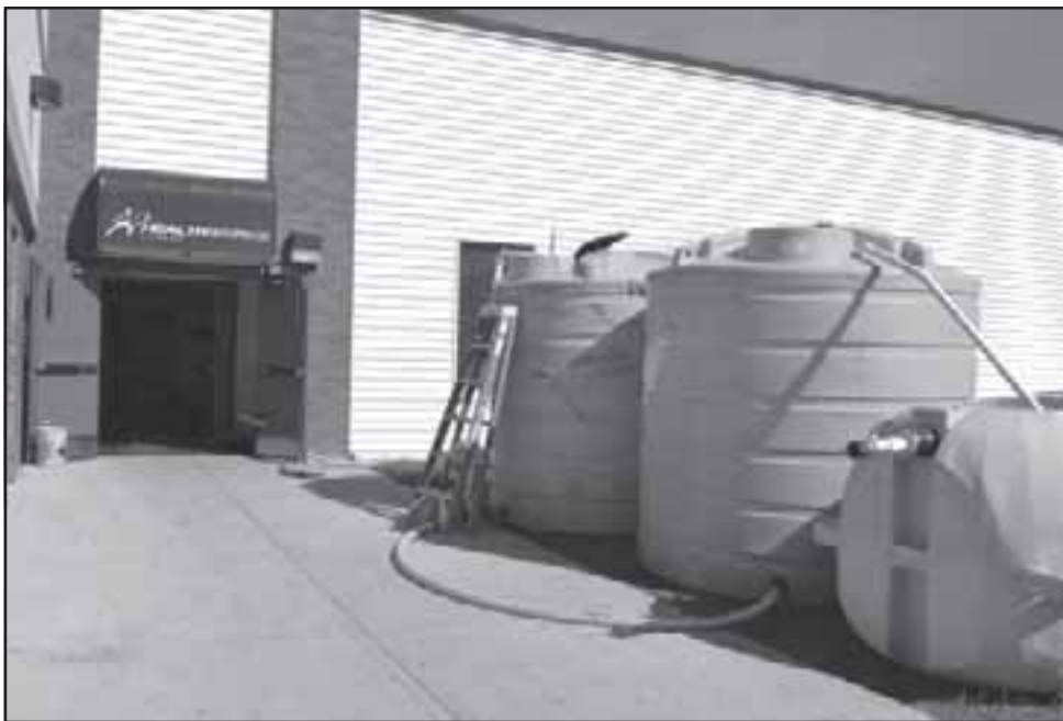
Waste water tanks are positioned in front of Healthworks with a hose that is pumping water out of the building.
