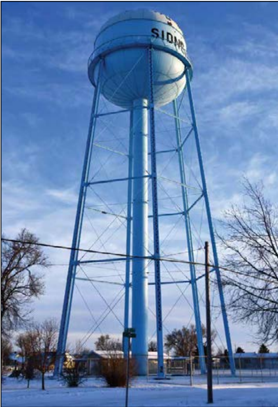
The current water tank at North Park (also known as Water Tower Park) in Sidney.
