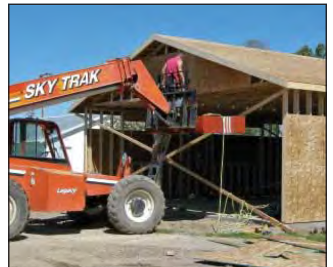
The booth during construction.
